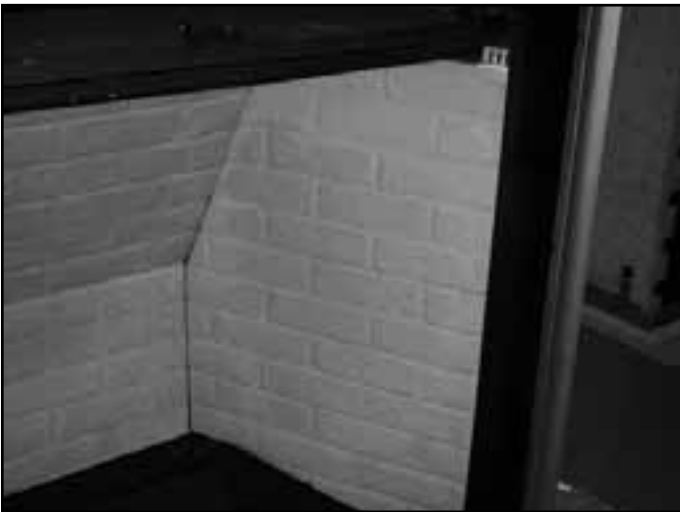
Figure 14.5 Install Right Side Refractory
